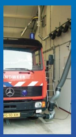
For exhaust extraction from emergency vehicles, we have an automatic disconnect. The hose stays attached to the vehicle tail pipe, then automatically disconnects at the door when vehicle exits the building. We offer the Euro-Track with electromagnetic disconnect nozzles and the Euro-Air-Track with pneumatic disconnect nozzle. We also offer simple mechanical nozzles for vehicles with overhead tailpipes.
